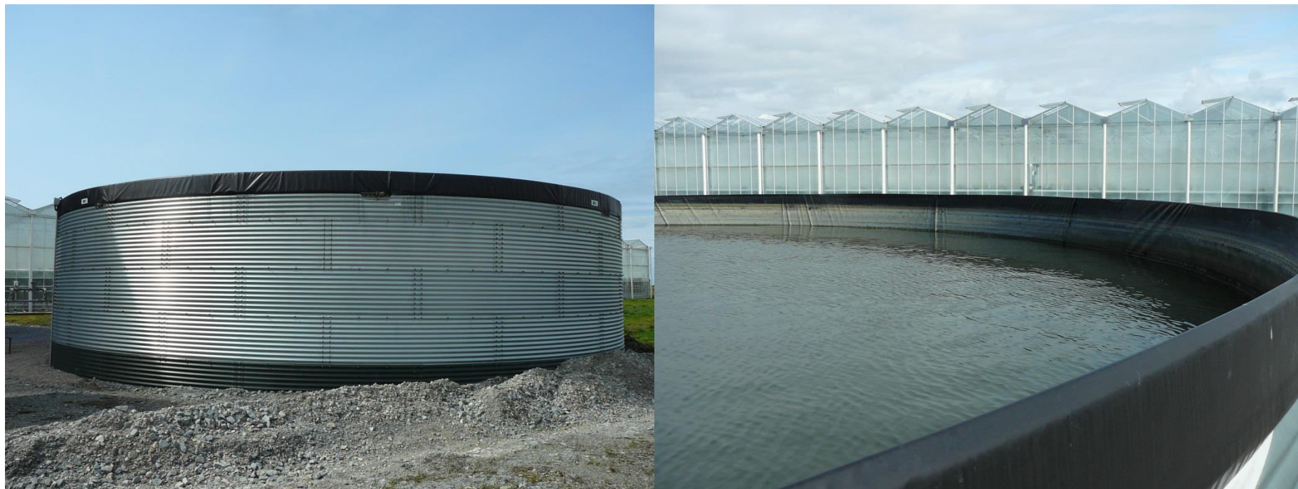
City water storage tank
