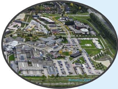
Hospital Waste Water Sneek
