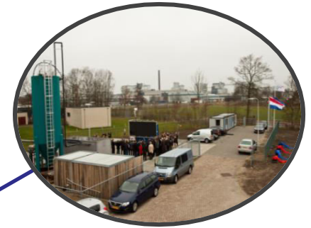
Municipal Waste Water Wetterskip Leeuwarden
