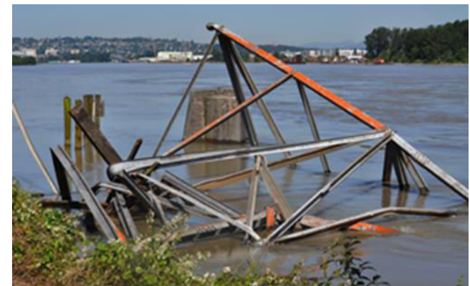
230kV line undercut by high river
